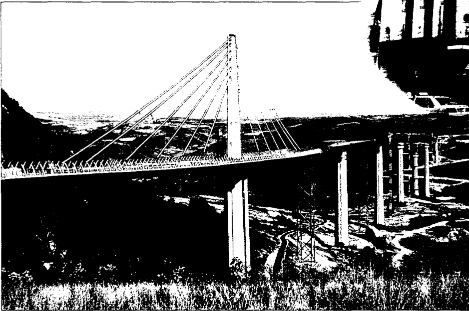
Millau Viaduct | Enerpac is a key partner in the construction of the Millau Viaduct in southern France. Our engineered hydraulic systems lift the temporary piers (seen in red) and push and align the 2.45 kilometer steel deck into place.
